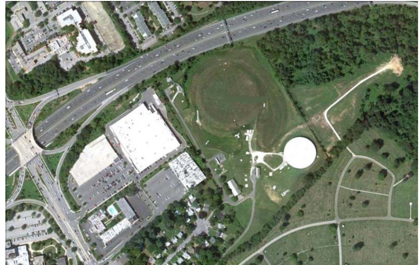
Existing Pikesville Covered Reservoir
